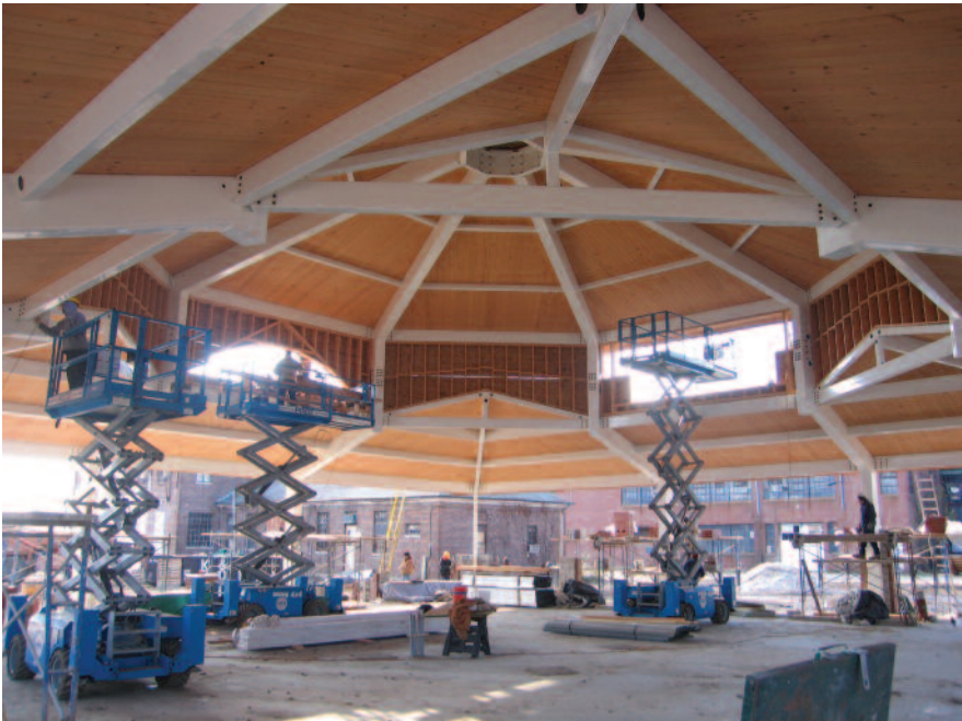
Extreme Powder Coating processed four semitrailer loads of steel for the carousel shelter.
