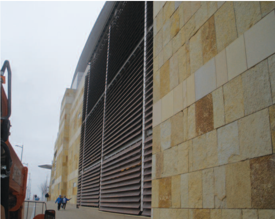
Target Field, home of the Minnesota Twins Baseball Team, sports powder-coated brackets processed at Extreme Powder Coating.
