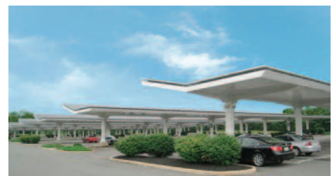
Keystone powder coated the structural steel used on this solar parking canopy designed and built by Solaire Generation.
